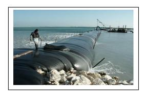
It is very resistant to microbial deterioration, chemicals, UV rays, and stress. It is less expensive than concrete or steel structures, easier to install, adaptable for a variety of terrain, non-polluting, aids in wetlands and coastal restoration, and is efficient in flood control, riverbank fortification, sludge dewatering, and landfill containment.
