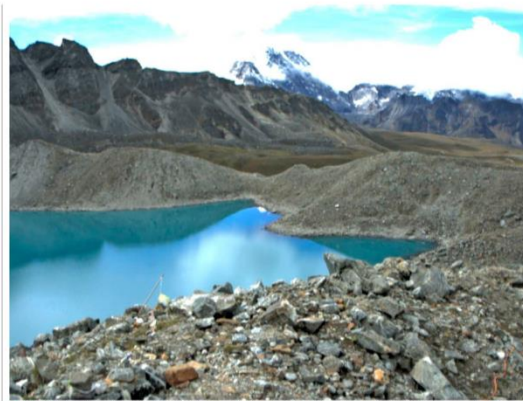
Definite risk: The south end of the Shaka Cho lake (5,200 m) in north Sikkim. The south end shows the weak debris that forms its moraine dam. www.issflood.org
