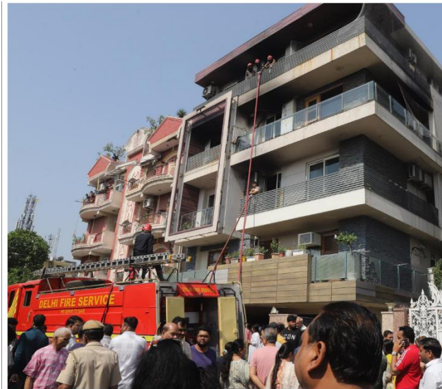
Tragic aftermath: A four-storey building in Vivek Vihar, where at least nine people died and two others were injured in a fire that broke out on May 3, 2026. SHIV KUMAR PUSHPAKAR
