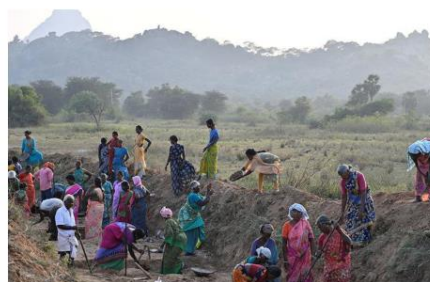
Right to work: People employed under the MGNREGA scheme dig a trench in Tiruvannamalai, Tamil Nadu. C. VENKATACHALAPATHY
